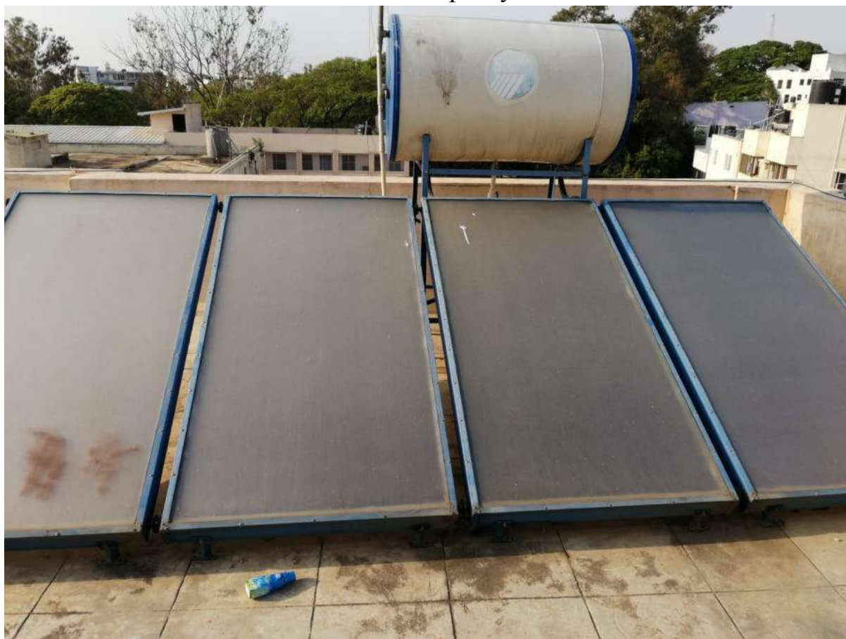
The solar water heater on the hostel building
